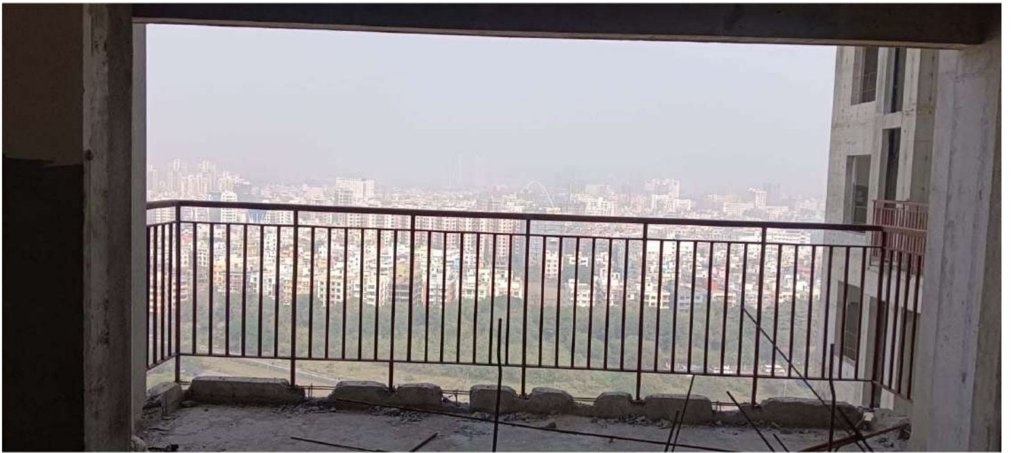
Tower 2 Balcony railing work
